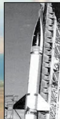
The Doorknob was a sounding rocket manufactured from Lacrosse rocket motors for the project Hardtack Nuclear Test Series.
